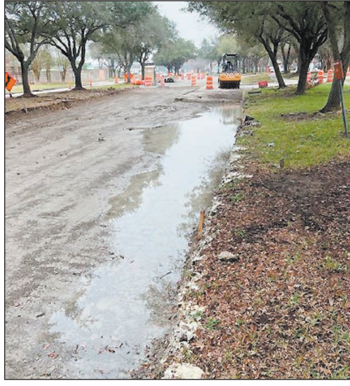
Bay Area Blvd project has been delayed by wet weather conditions
